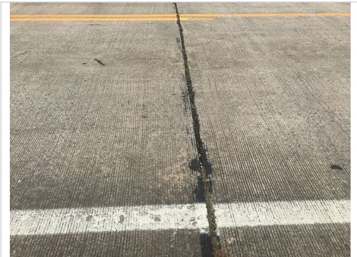
Joints missing seal.
