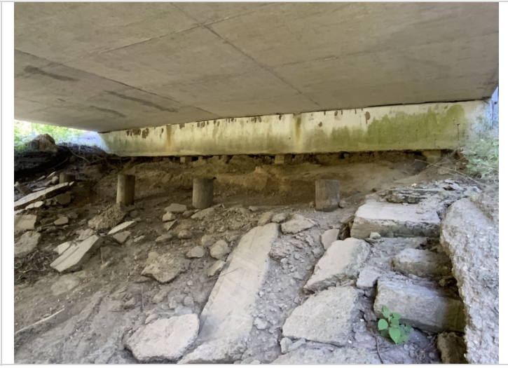
Abutment 2 erosion under cap exposing pile.
