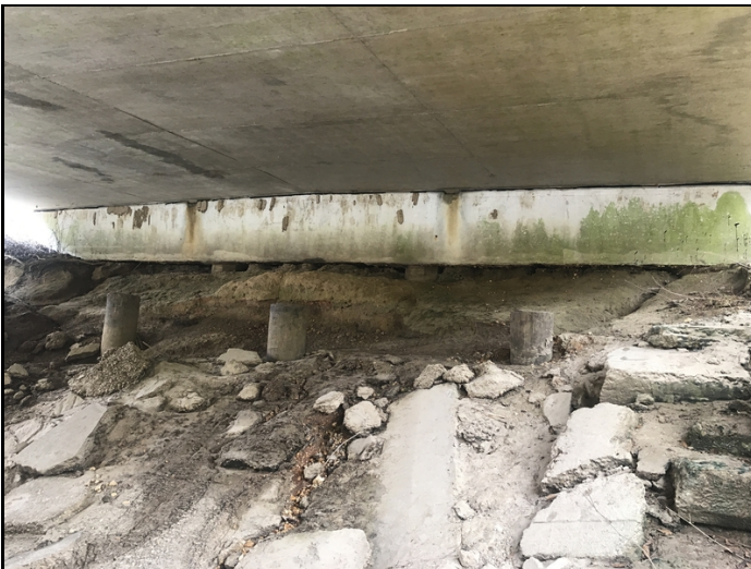
Abutment 5, erosion under cap.
