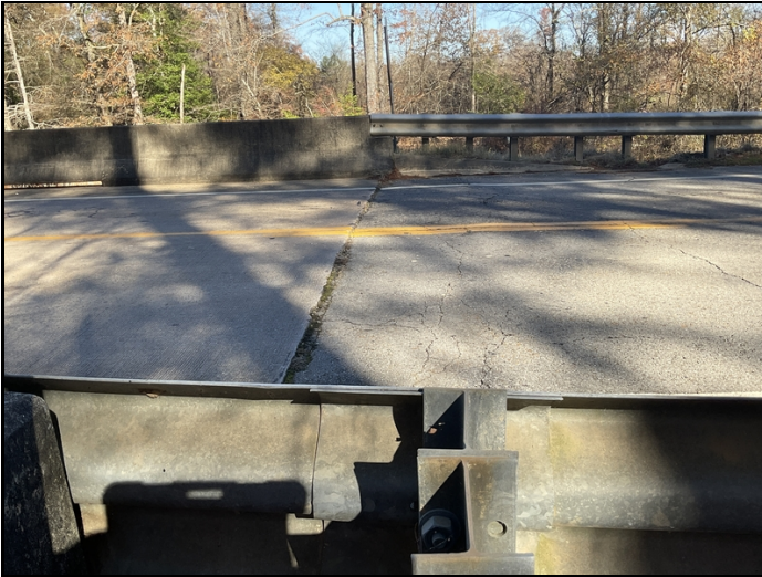
Roadway settlement abutment 2
