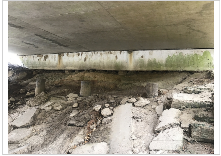
Abutment 5, erosion under cap.
