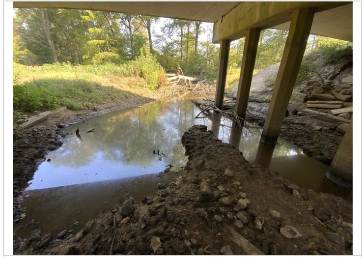
Bent 4 has scour hole up to 1'6"
