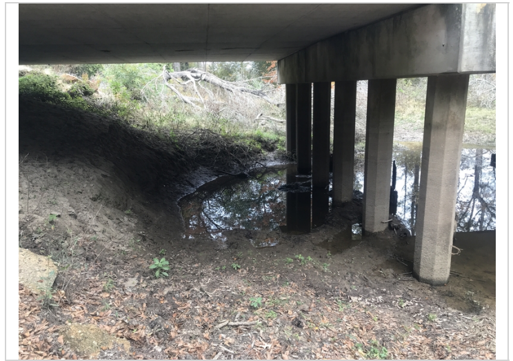
Span 1, erosion to slope, minor scour around bent 2.
